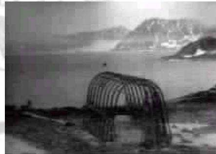
Camp Wellman, Virgo Bay, Danes Island, Spitsbergen, showing the 1906-07 hangar under construction
